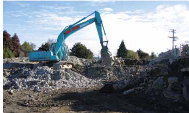
Remediation work at FCC site
