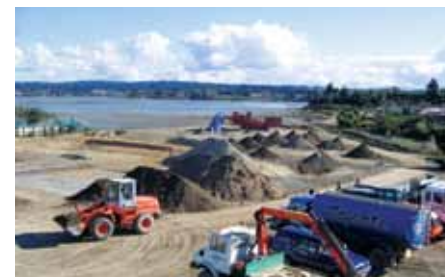
Remediation site works
